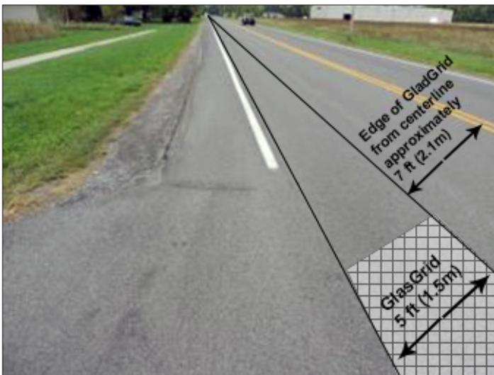
(Fig. 5) Crack from edge of roadway is present across the shoulder area however it ends where the GlasGrid® is located
