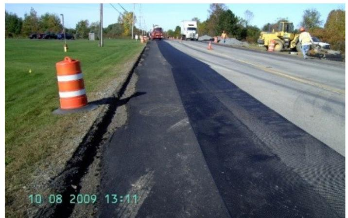
(Fig. 4) Placement of GlasGrid® in preparation of the new wearing course.
